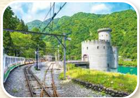
Yanagibashi Station• Shin-Yanagawara Power Plant
